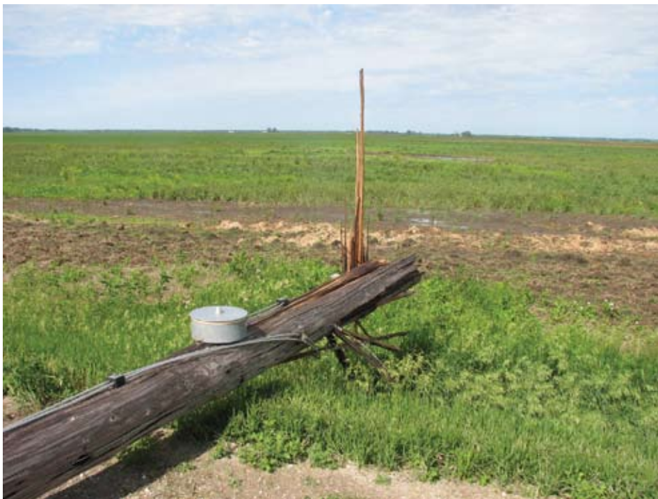
This is one of 23 NIPCO poles damaged when strong winds and a tornado swept through Harrison and Monona counties on June 11. While the poles were snapped off, the conductor remained unbroken.
