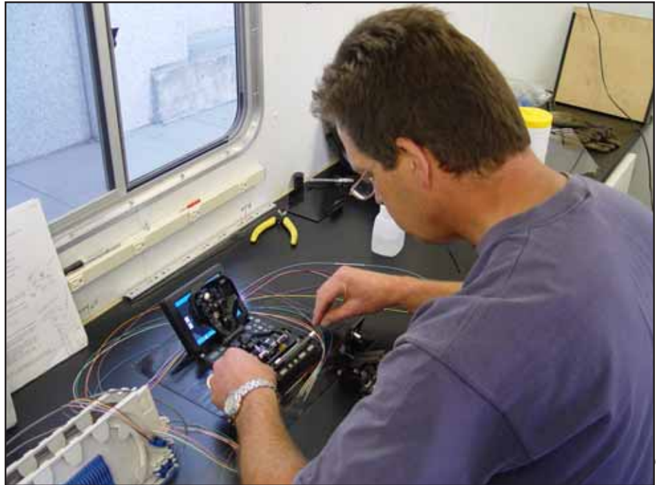
Senior telecommunications technician Keith Schiltz splices fiber optic cable in NDC's fiber trailer.
